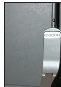
Door leaf is prepared for the Exidor 294 panic bolt
