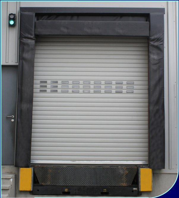
Dock Leveller Installation
